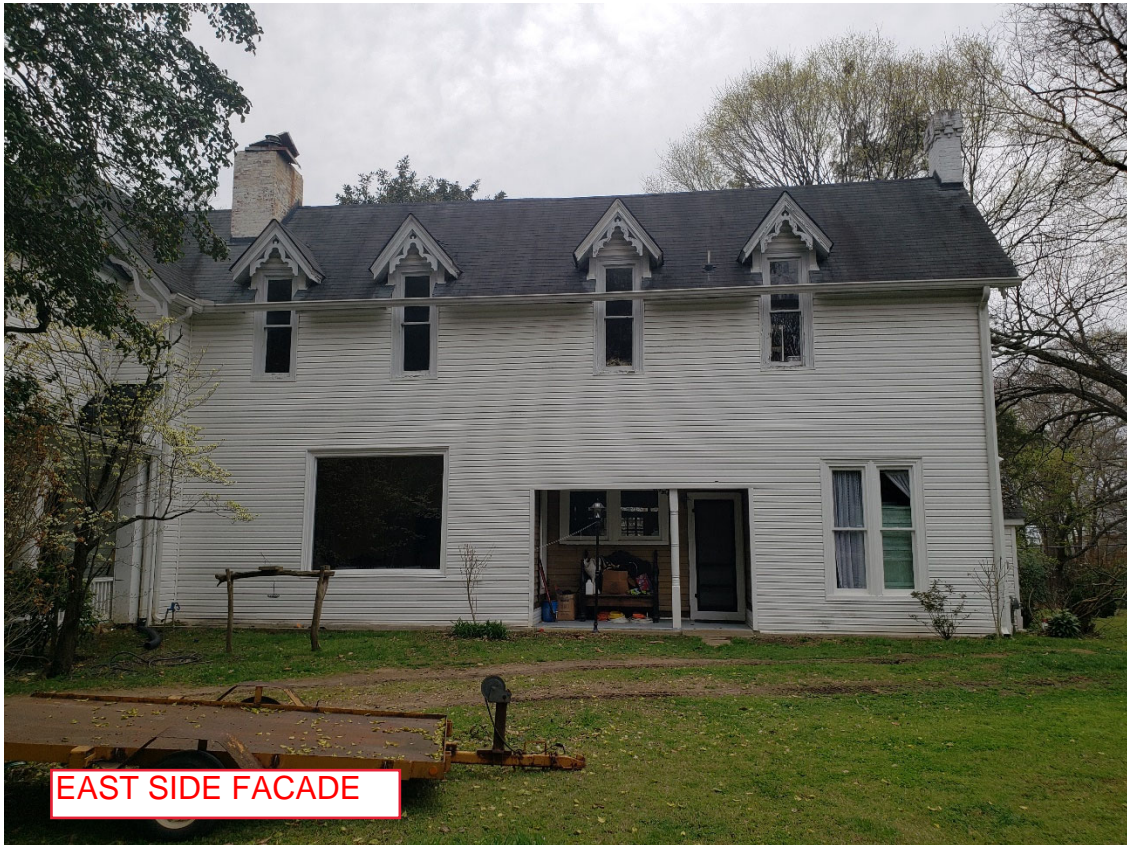
EAST SIDE FACADE, FRONT PORCH
