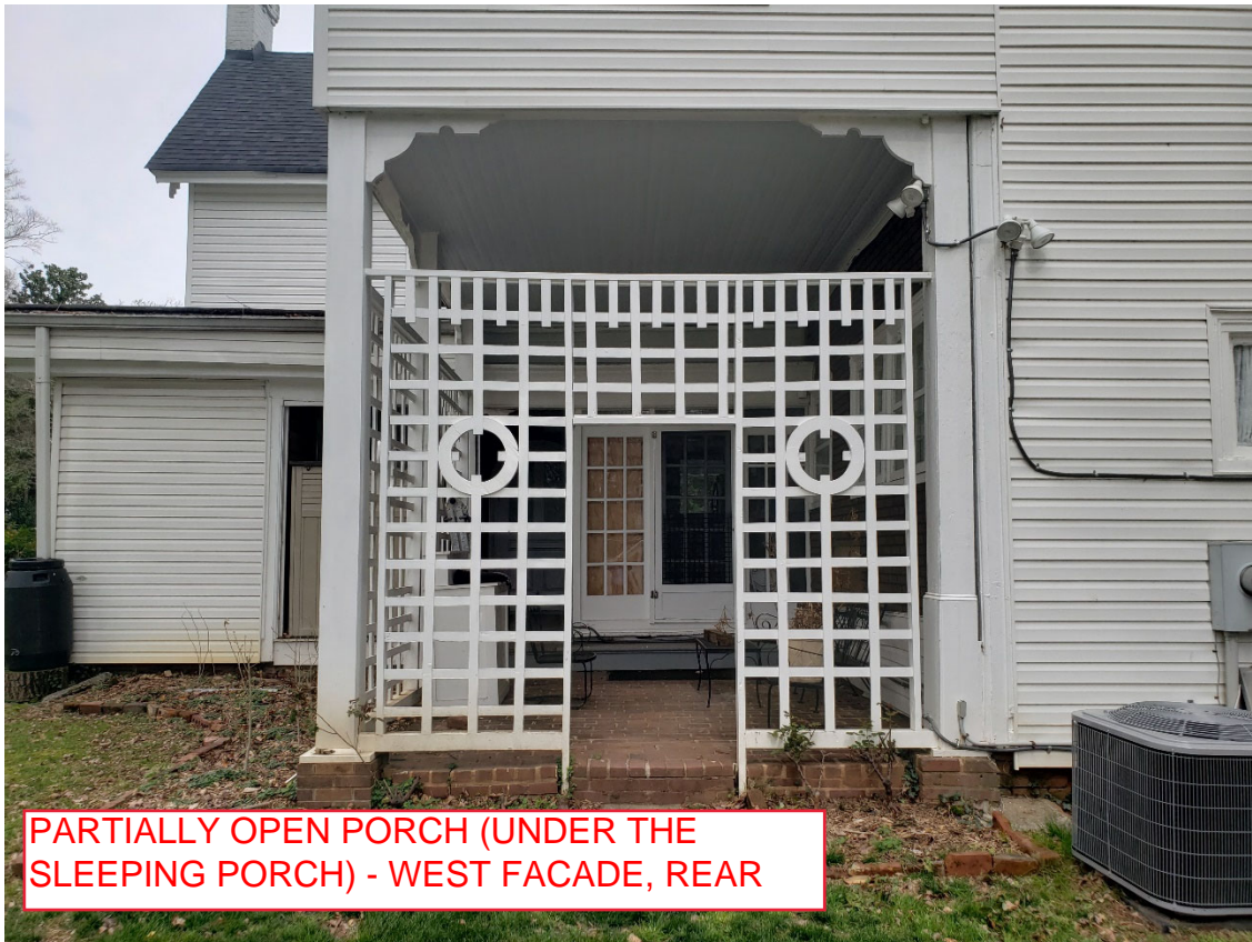
PARTIALLY OPEN PORCH - WEST FACADE, REAR
